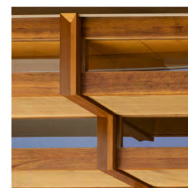
1. TIMBER CANDALEPAS ASSOCIATES - LITTLE SISTERS HOUSE
